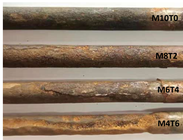
Figure 4.5.3. Surface morphology of reinforcement in mortar specimens at the end of accelerated corrosion.
