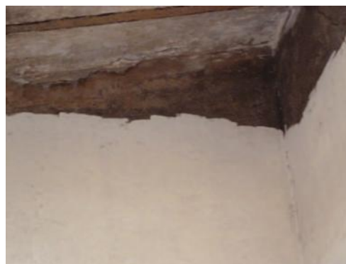
F-MAT-004 MURO INTERIOR
