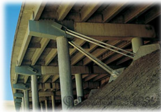
Figura 1.17 Rehabilitación en los cabezales (Tomada de http://www.dsiamerica.com/products/repair-strengthening/seismic-upgrading/bartendons/elisian-viaduct-la-usa.html )
