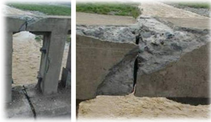
Figura 1.5 Golpeteo en la estructura del puente (Tomada de http://www.fhwa.dot.gov/publications/research/infrastructure/structures/11029/003.cfm )
