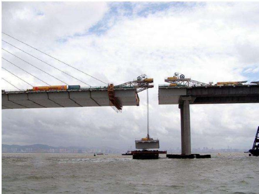
Figura 1.9 Voladizos sucesivos (Tomada de Construction engineering of the hongkong-shenzhen cable-stayed bridge.)
